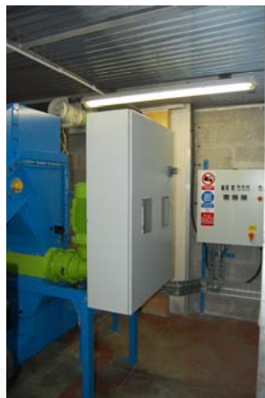
System and shredder Controls
