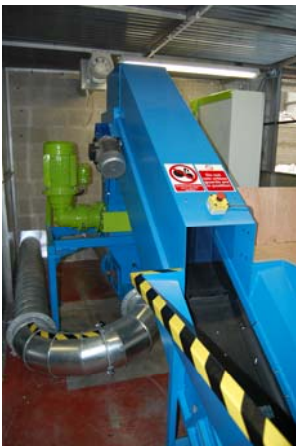
Bulk hopper and conveyor
