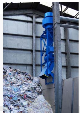
Cyclone and rotary valve discharge
